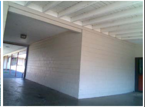
SW Primary Structural Type
