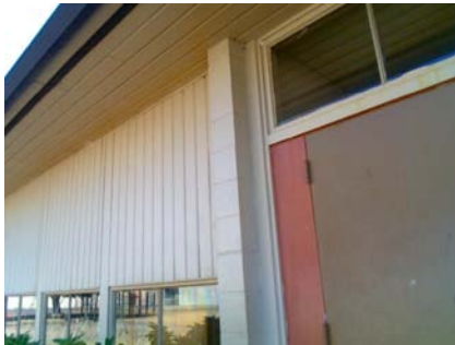
N Primary Structural Type
