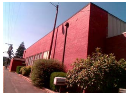
S Seismic Upgrade BOLT HEADS AT ROOF LINE
