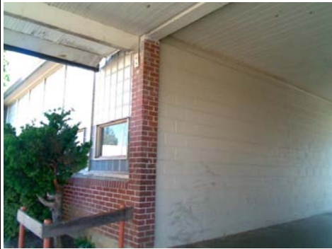
SW Primary Structural Type
