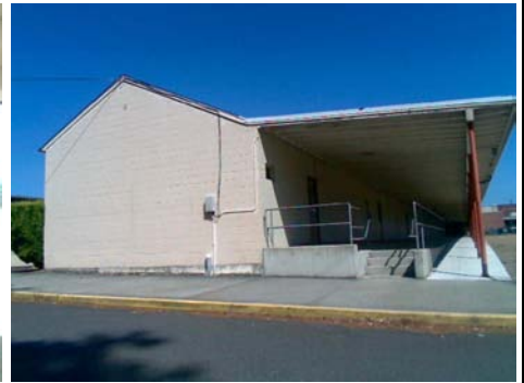
SW Primary Structural Type
