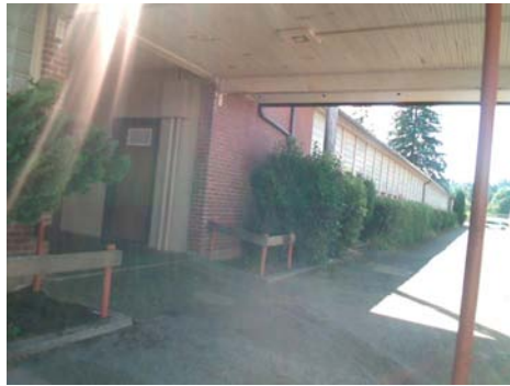
NE Elevation View
