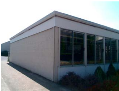
NE Primary Structural Type cmu endwall
