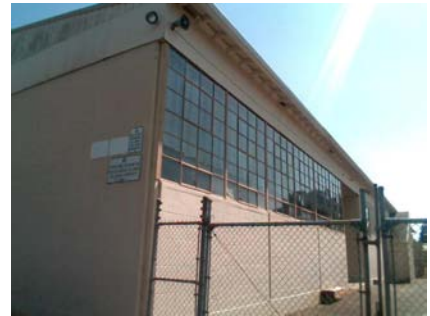
W Plan Irregularity Tertiary SKINNY STL COLS IN WINDOW BANK ALL ALONG W SIDE
