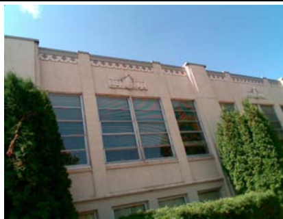
E Poor Condition pour line at top of windows
