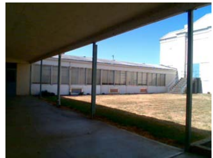
E Primary Structural Type both w and cmu
