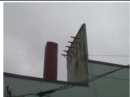
N Falling Hazard Unreinforced chimney and tall concrete wall (> 6 ft)
