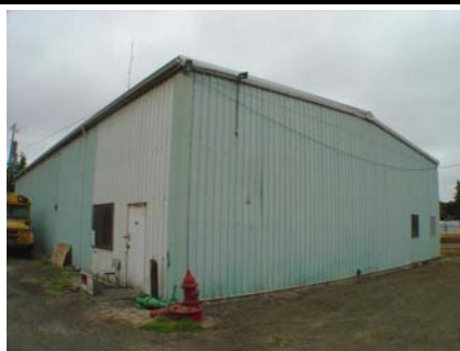
NE General Site
