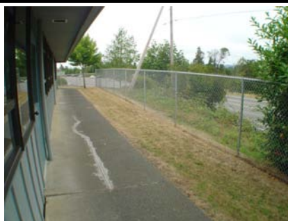
E Other Walkway is settling towards HWY 101 which is at a lower elevation.
