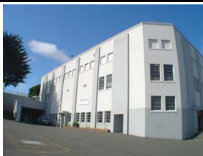
NE Vertical Irregularity Primary Two stories vs. one in the first picture. It looks like three floors but the "two top floors" are the gym.
