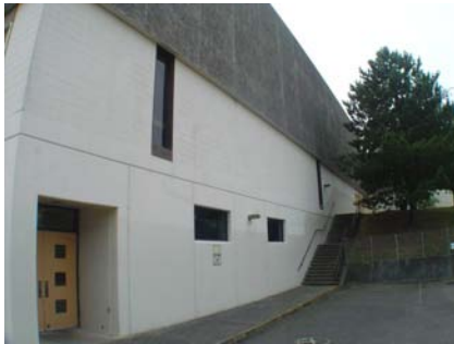
NE Vertical Irregularity Secondary sloped site
