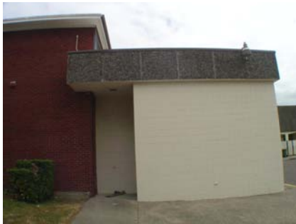
W Vertical Irregularity Tertiary
