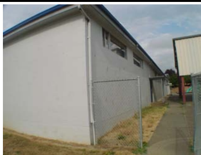
SW General Site
