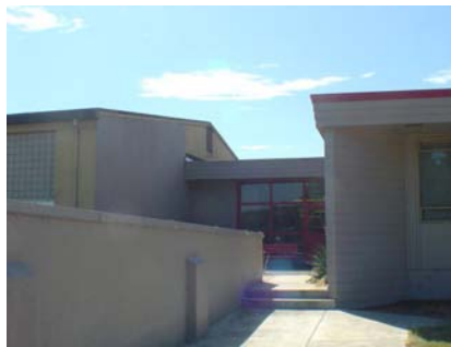
NE Vertical Irregularity Primary
