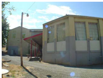
E Plan Irregularity Secondary This is very small compared to the size of the building.
