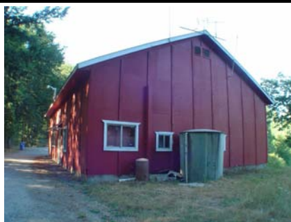
SW General Site
