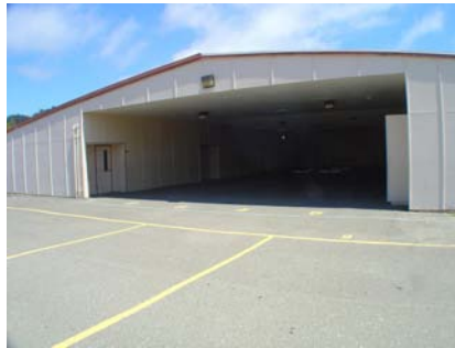
N Plan Irregularity Tertiary All 3 legs of this building have a very large and deep opening.
