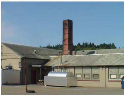
E Falling Hazard This is partially-reinforced
