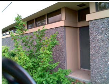
NW Primary Structural Type inconclusive wall construction
