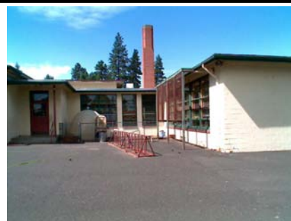
S Falling Hazard
