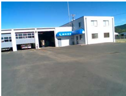
W Vertical Irregularity Primary also shows a reentrant corner.
