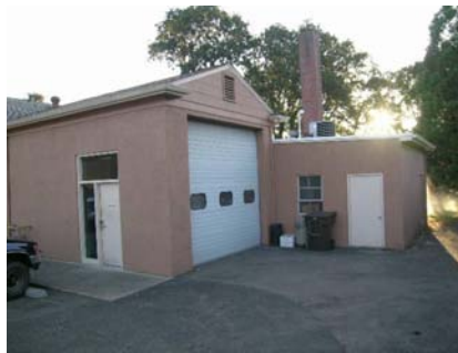
SW Falling Hazard also step in elevation and reentrant corner
