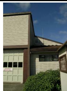
E Primary Structural Type and secondary structure type, RM on the bot. garage wall and W2 above.
