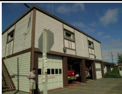
SE Plan Irregularity Secondary Large openings, the back wall of this garage is solid RM indicating a potential Torsion problem.
