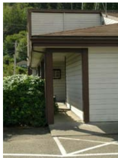
NE Plan Irregularity Primary Out of plane lateral system and an elevation step.
