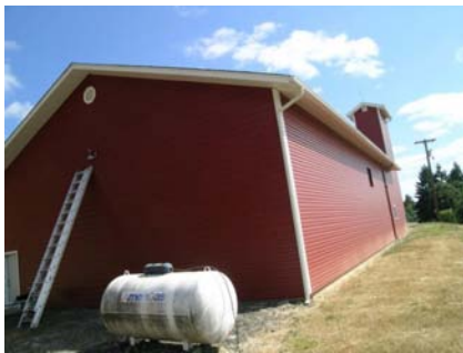
NW Vertical Irregularity Primary due to hose tower
