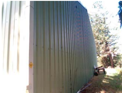
N Plan Irregularity Primary backwall solid indicating torsion problem
