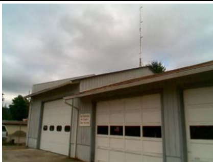
SE Vertical Irregularity Primary
