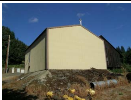
SW Plan Irregularity Primary back wall is solid indicating a possible Torsion problem.
