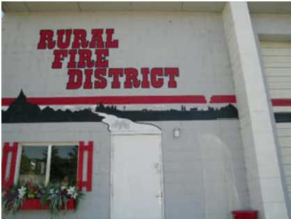
N Primary Structural Type
