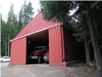
SW Elevation View
