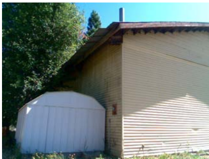
SW Plan Irregularity Primary back wall is solid: Torsion
