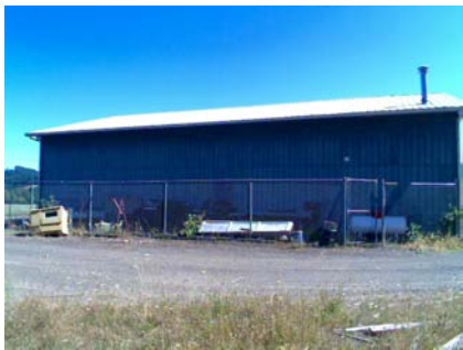
N Plan Irregularity Primary back wall is solid indicating a potential torsion problem.
