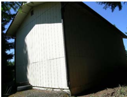
SE Plan Irregularity Primary back wall is solid indicating a possible torsion problem.
