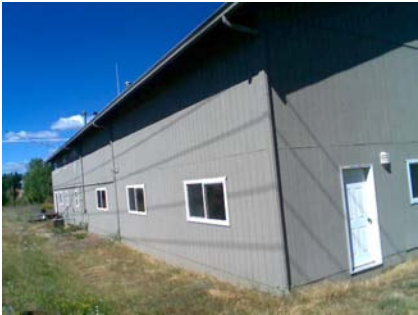
SW Plan Irregularity Primary back wall is solid indicating a potential torsion problem
