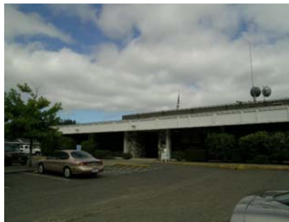
S Vertical Irregularity Primary raised S3 section that gives the building increased head height through the center of the building. Thus, this irregularity also creates a large opening.
