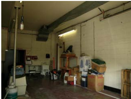
SE Secondary Structural Type RM walls on the sides and back of the garage form a "C" shape indicating a potential torsion problem.
