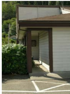
NE Plan Irregularity Primary out of plane lateral system and elevation step.
