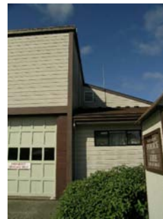
E Primary Structural Type and secondary structure: RM wall on the edge of the garage wall and a W2 wall above.
