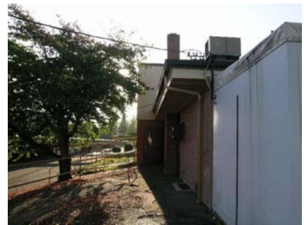
W Falling Hazard Reinforced chimney? and out-of-plane offset
