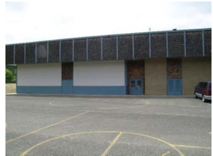
NE Primary Structural Type and secondary structural type. The wall on the left is W2 and the wall on the right is RM.
