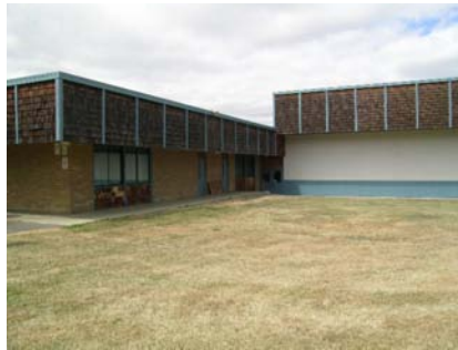
SE Primary Structural Type secondary structure type, reentrant corner, elevation step.
