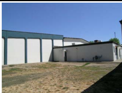
SW Vertical Irregularity Primary and reentrant corner
