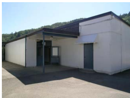
NW Vertical Irregularity Primary and reentrant corner
