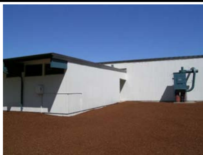
SE Plan Irregularity Primary and step in elevation
