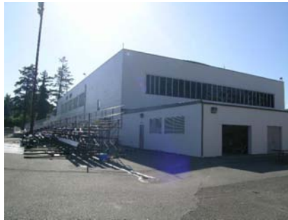
NW Vertical Irregularity Secondary
