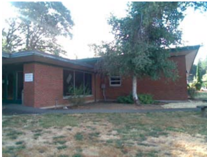
NW Plan Irregularity Primary reentrant corner
