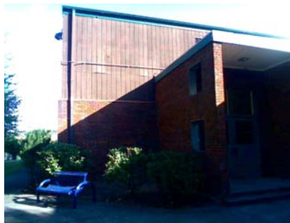
S Secondary Structural Type W2 at the upper level
