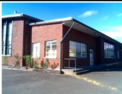
NE Plan Irregularity Secondary and elevation change
