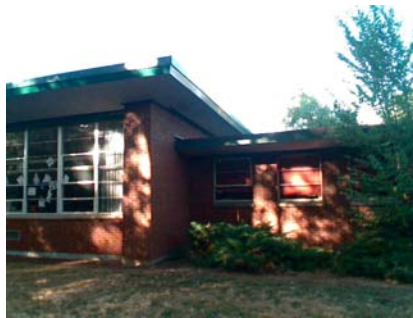
NE Vertical Irregularity Primary and reentrant corner.
