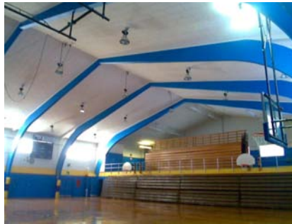
E Primary Structural Type large wood arches
