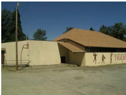
S Vertical Irregularity Primary and reentrant corner
