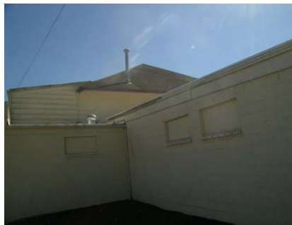
NE Vertical Irregularity Primary and reentrant corner
