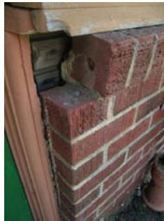
N Primary Structural Type wood behind façade.
