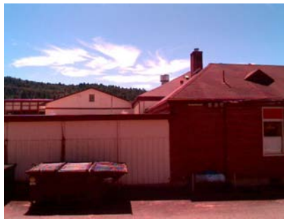
N Vertical Irregularity Primary building A is on the right, B is on the left. Also shows URM chimney.
