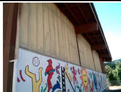
W Secondary Structural Type plastic on the upper section of this wall.
