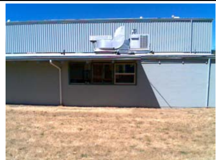
S Vertical Irregularity Primary also shows RM1 for the lower level and S3 for the upper level.
