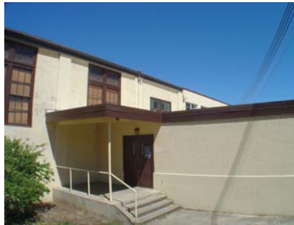
S Plan Irregularity Tertiary step in elevation with adjacent bldg
