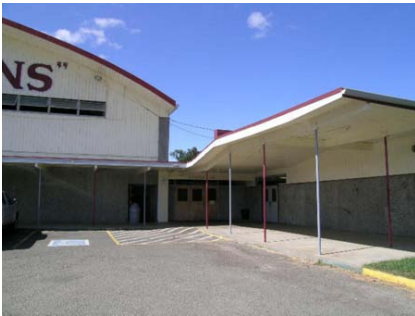
SW Vertical Irregularity Secondary and reentrant corner due to adjacent building. Building A is on the right and building B is on the left.
