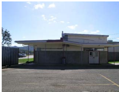
E Vertical Irregularity Secondary and reentrant corner.
