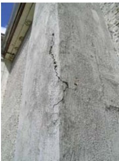
W Poor Condition cracked concrete column. There is also evidence of concrete spalling that has been patched.
