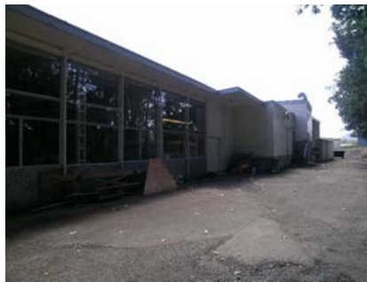
NW Plan Irregularity Tertiary out of plane LFRS
