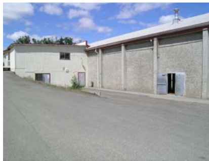
SW Vertical Irregularity Primary sloped site and reentrant corner. The top half of the left section is W2.
