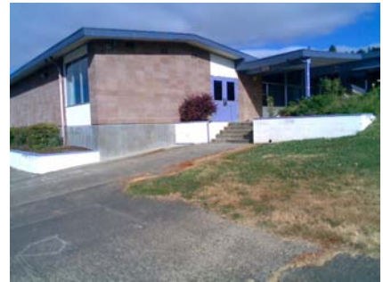
SE Vertical Irregularity Primary sloped site
