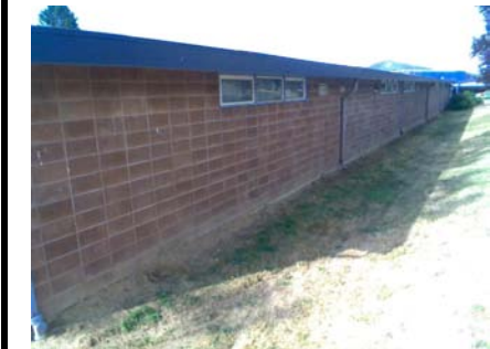
N Plan Irregularity Primary solid back and ends, open front
