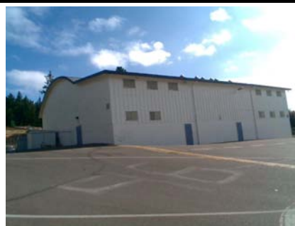
S Vertical Irregularity Secondary sloped site (minor)
