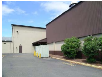
SE Plan Irregularity Secondary reentrant corner due to adjacent building. Building A is on the left and building C is on the right.
