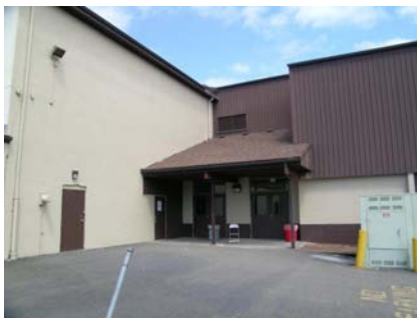
SE Plan Irregularity Secondary due to adjacent building. Building A is on the left and building C is on the right.
