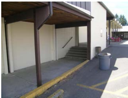
NE Vertical Irregularity Primary
