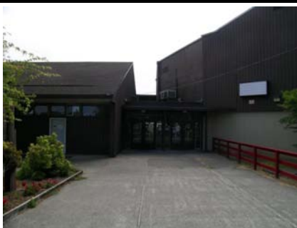
NE Vertical Irregularity Secondary and secondary plan irregularity building A is on the left and building B is on the right.
