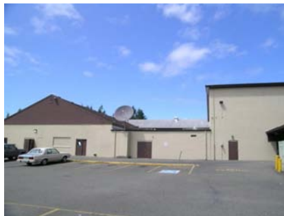
SW Vertical Irregularity Primary
