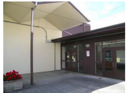
SW Vertical Irregularity Primary and reentrant corner
