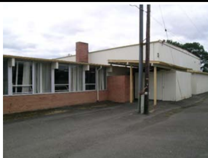
NE Vertical Irregularity Primary and reentrant corner
