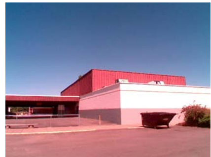
SW Primary Structural Type and secondary structural type. W2 is on the upper level and RM is on the lower level.
