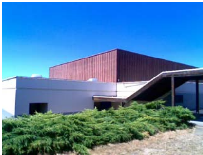
SE Vertical Irregularity Primary and reentrant corner
