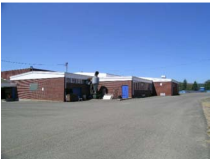
SE Plan Irregularity Primary and step in elevation
