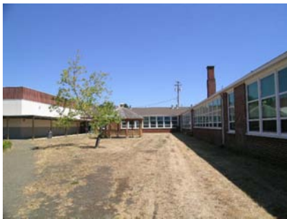
NW Falling Hazard and reentrant corner
