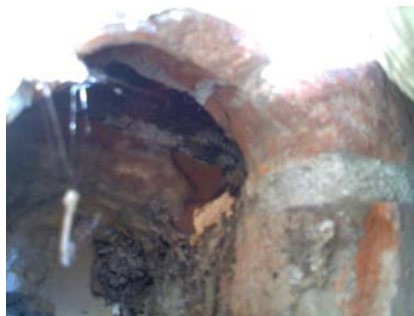
S Secondary Structural Type PIC OF HOLE IN BRICK
