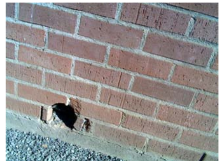
S Secondary Structural Type 2ND WYTHER OF BRICKS IN HOLE AND A ~2" GROUTED CAVITY
