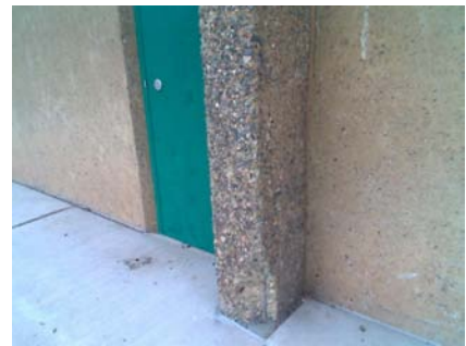
SW Other poor concrete
