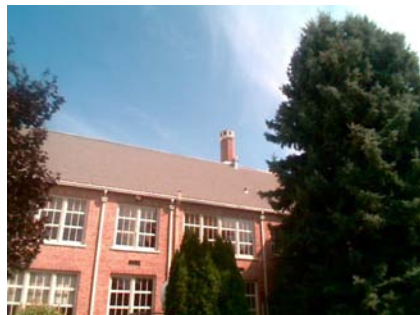
S Falling Hazard smokestack
