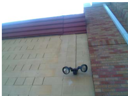
W General Site cracks from eq
