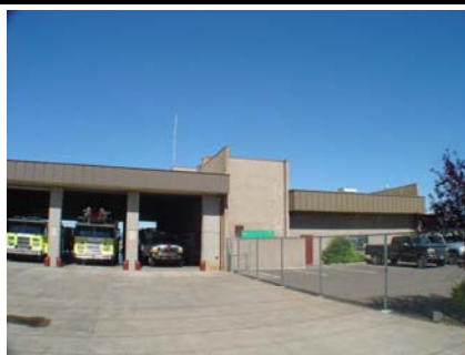
W Vertical Irregularity Primary Also shows large doors on both sides of the building indicating that there is not a torsion problem.
