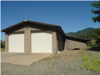
W Plan Irregularity Primary Shows garage doors on both sides indicating that there is not a torsion problem.
